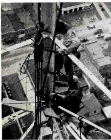
TOP MEN in their profession are Eddie Melley (upper figure) and Buddy Speir as they tighten bolts at 450-ft. level of WOR-TV New York's tower under construction at North Bergen, N. J. When completed, tower will be 760 ft. high.
